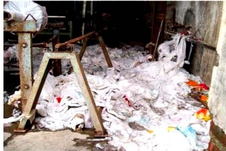
Garbage inside a factory
