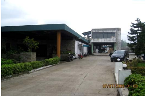
Factory offices (left) and goods loading bay (right)
